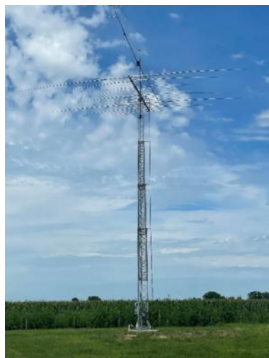
Figure 1 OB-12 Normally @60', 80m rot dip @'72'. K3S, Expert 2K amp and Green Heron Ro- tor Control in ranch house bedroom.
