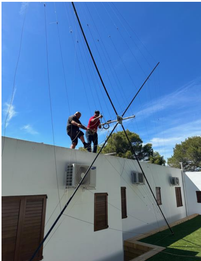
EA6AOV Josep and CO8NMN (#2082) Noe helping dismantle the antenna.
