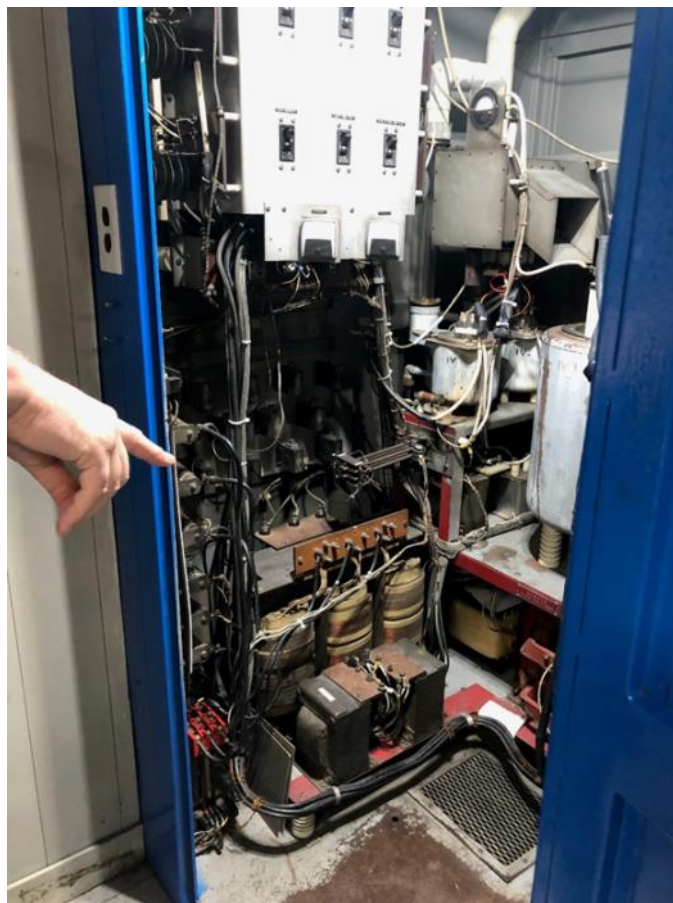
Glenn pointing at Modulator Cabinet for the GE 250KW transmitter.
