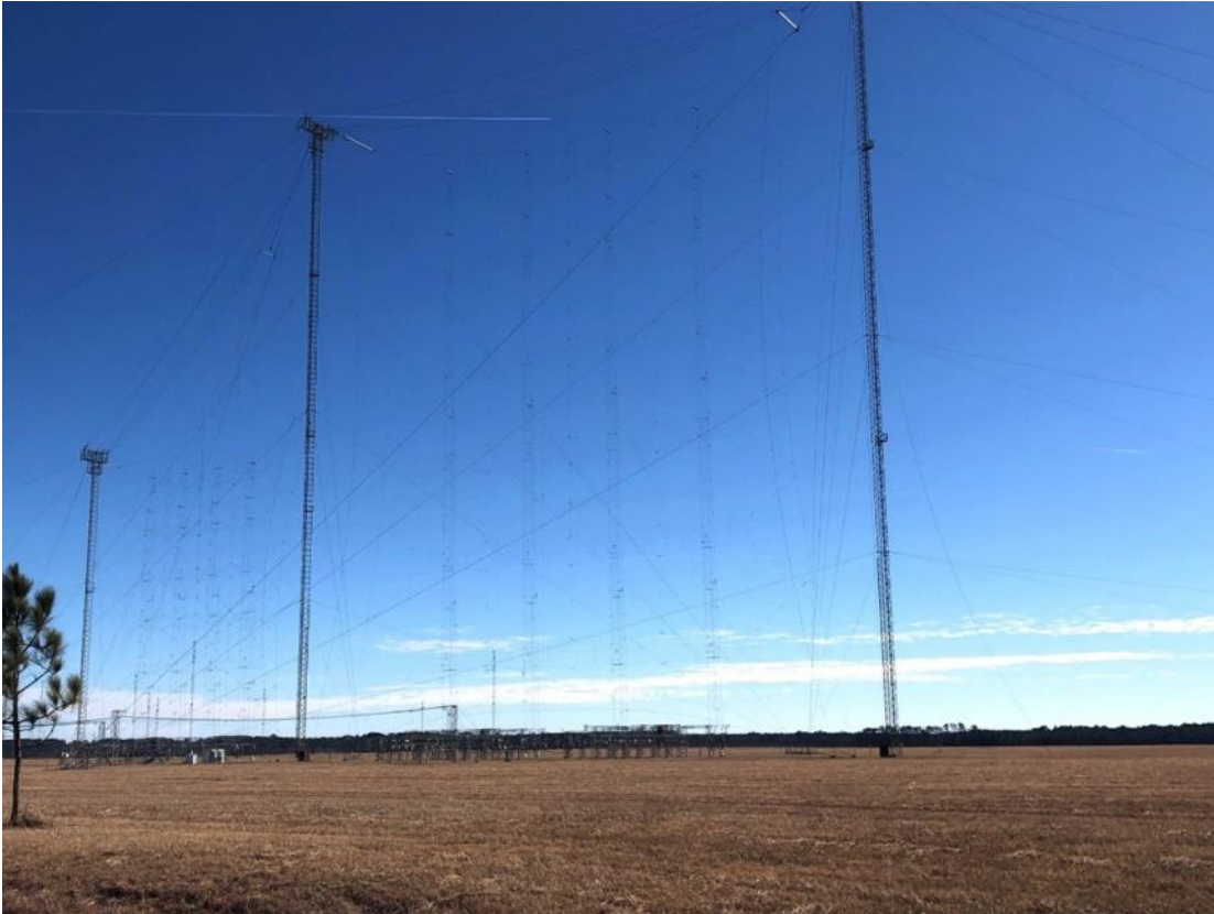
TCI "Curtain" antenna made of 4 dipoles wide & 6 dipoles high, pointed at Cuba. It is controllable in both vertical and horizontal azimuth, depending on the configuration has to up 23dB gain at a 4 degree take off angle.
