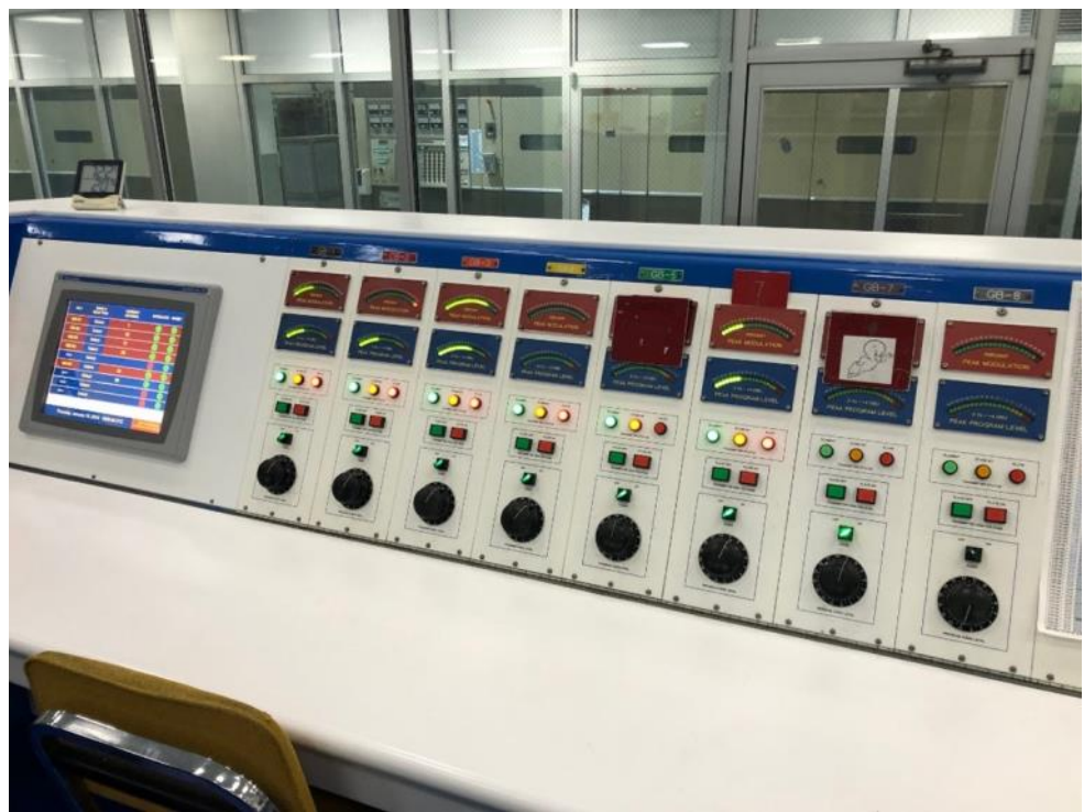
GB-6 Transmitter Monitor & switches.
