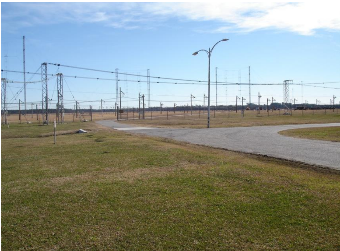
Curtain and Rhombic antennas fed from the antenna switching center.
