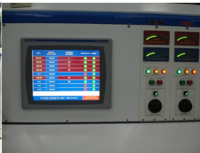
Antenna switch controller for matching the 8 transmitters with 38 antenna configs.
