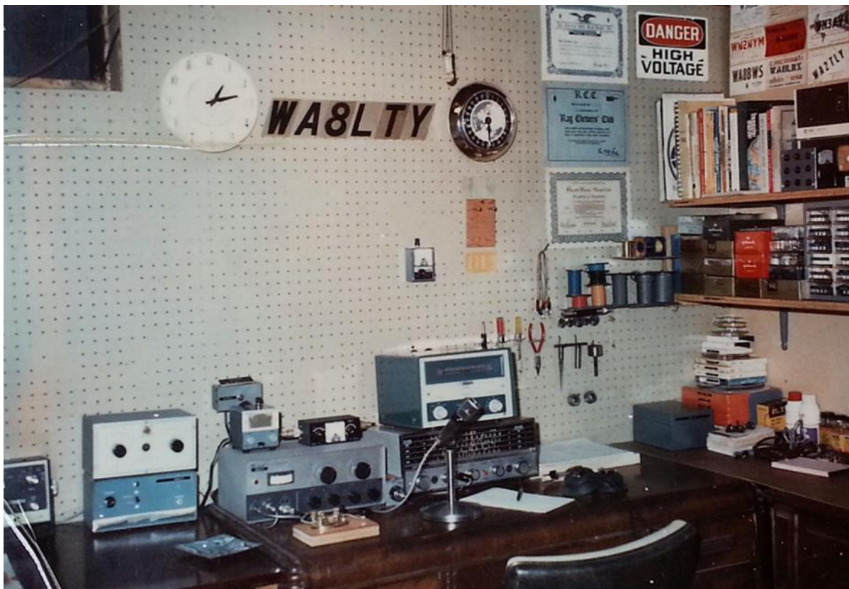
WN8TLY/WA8LTY Station 1964. 60 Watts, all tubes. CW and AM
