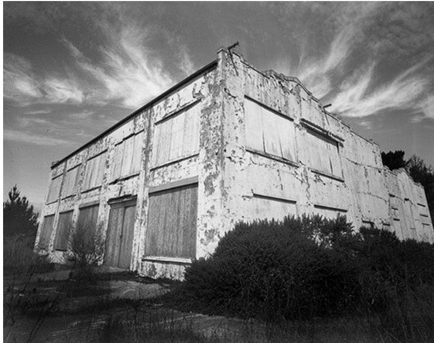
Here's what left of the Bolinas Building 1 where the Marconi station was installed in 1914.
