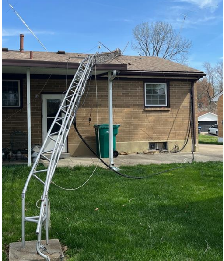
Tower damage at K4WW
