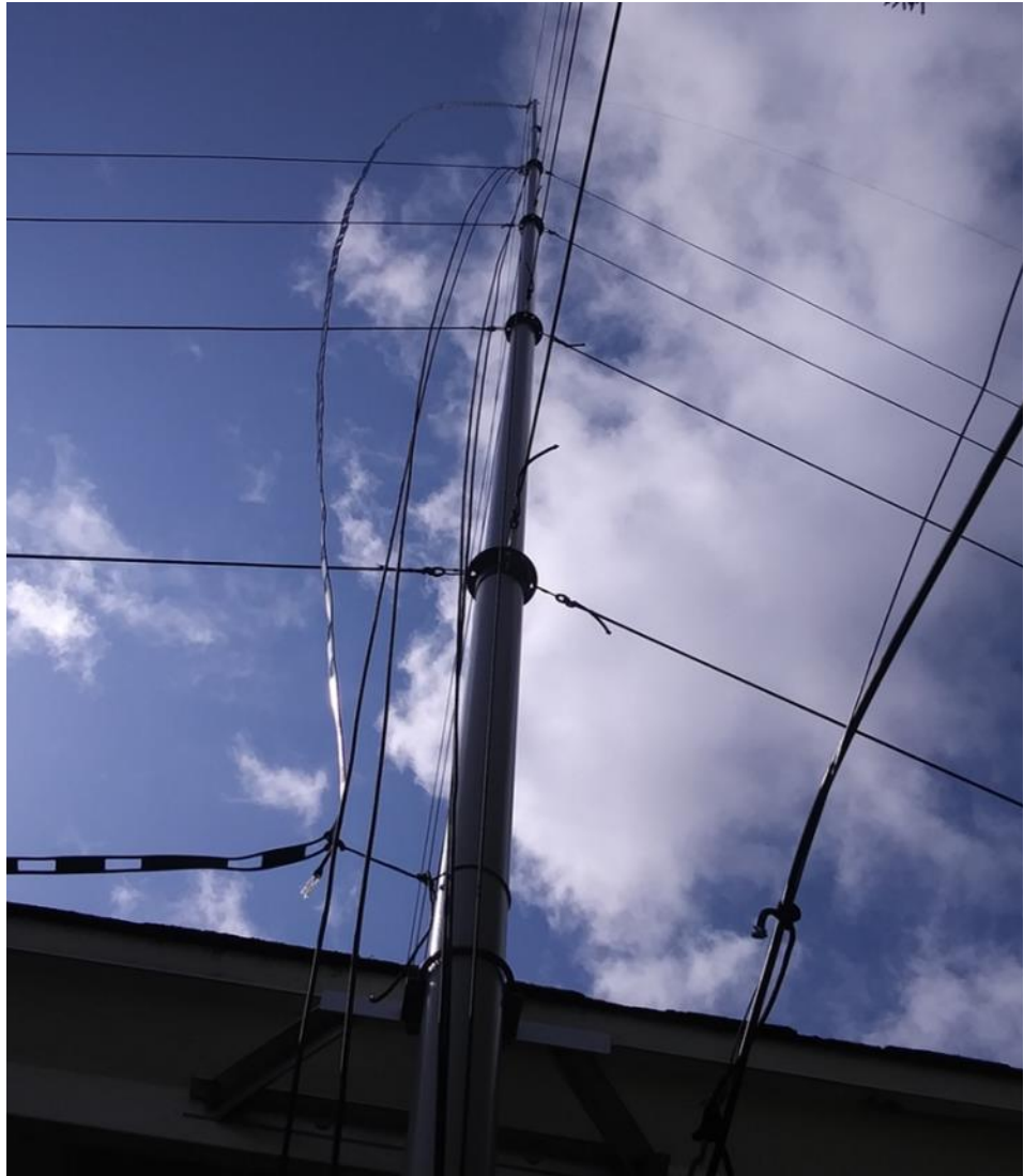
New mast at AB7MP
