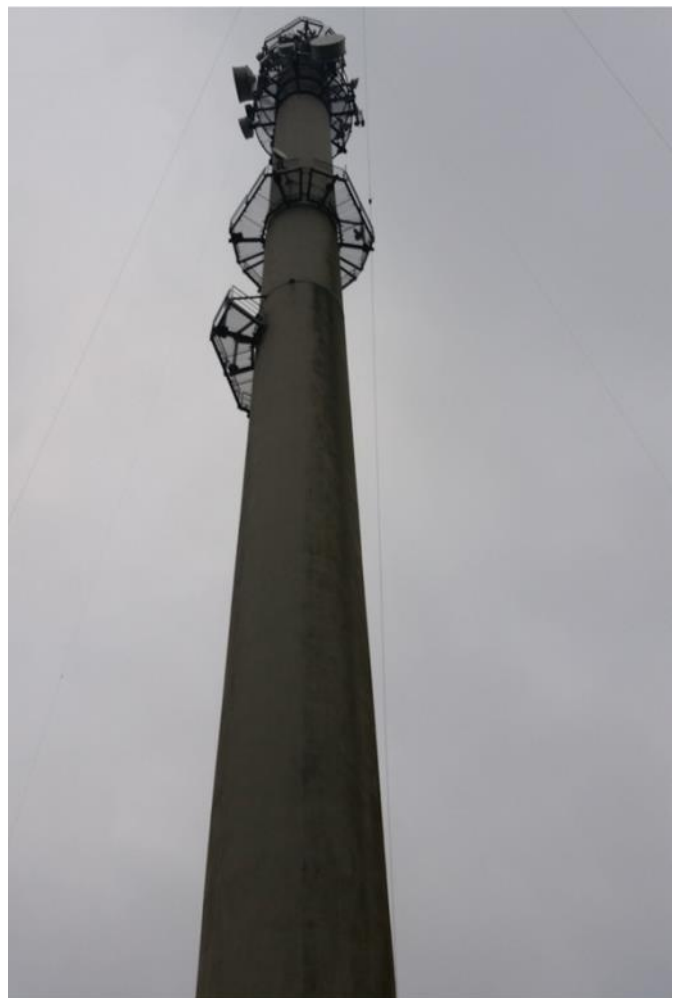
70 m tower from below
