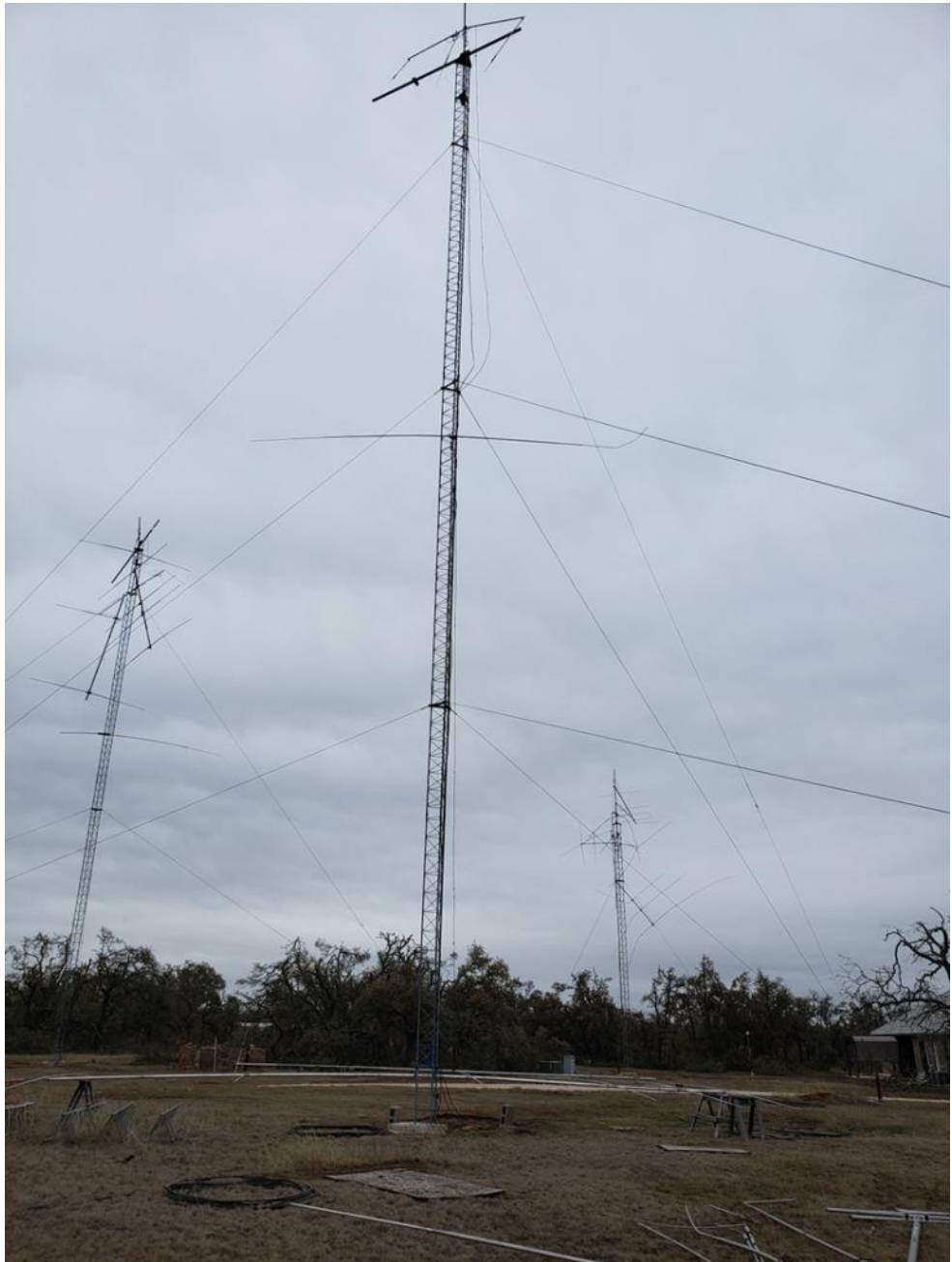
The aftermath - February 25, 2021 -- L-R: 15M Tower with broken 40M dipole at 50', 20M/WARC tower with only survivor - the 20M dipole at 50', and the 6M/Bencher SkyHawk tower. At the base of the 20M tower is a M2 6el 15M Yagi that was staged to go up on the 15M tower (to be the fixed on JA). Miraculously none of the falling boom/element pieces of the 5 element 20M Yagi (bottom right corner) hit it. Since this picture, the boom and 4 elements on the top right of the 15M tower has fallen to the ground. Note the back half of the Bencher Skyhawk on the right hand tower - hanging by a broken element that went through the tower rungs. Also, an example of the extensive tree damage. Note -- the fifteen meter tower is not really leaning - just a result of the wide angle photo lens.
