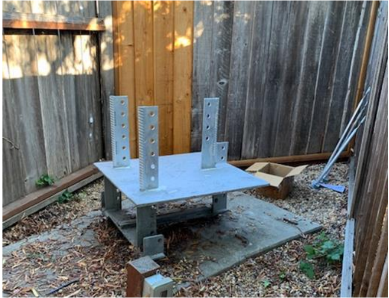
Custom mounting plate rests on top of existing base
