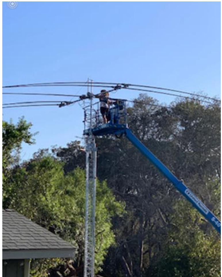
Mounting the DB18 using a 40-foot boom lift
