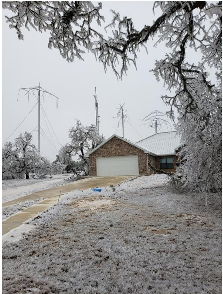
February 13, 2021 – 3 days into the freeze: L-R: 5el 20M/WARC Tribander on 100' (32 meters) tower; 222 & 432 Yagis on 47' (15 meters) tower; 7 el 15M Yagi and 5 el 6M Yagis on 90' (28 meters) tower (mast is now bent); 7el 6M LFA/12 el 2M/Bencher SkyHawk/5 el 6M Yagi on 50' (16 meters).
