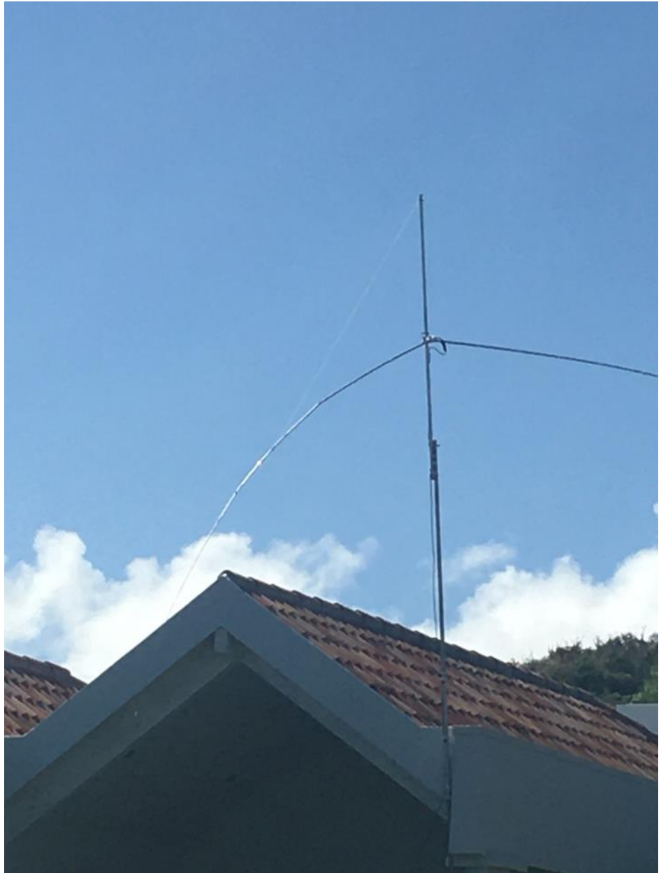
Our sad 20 m dipole after a wind storm .
