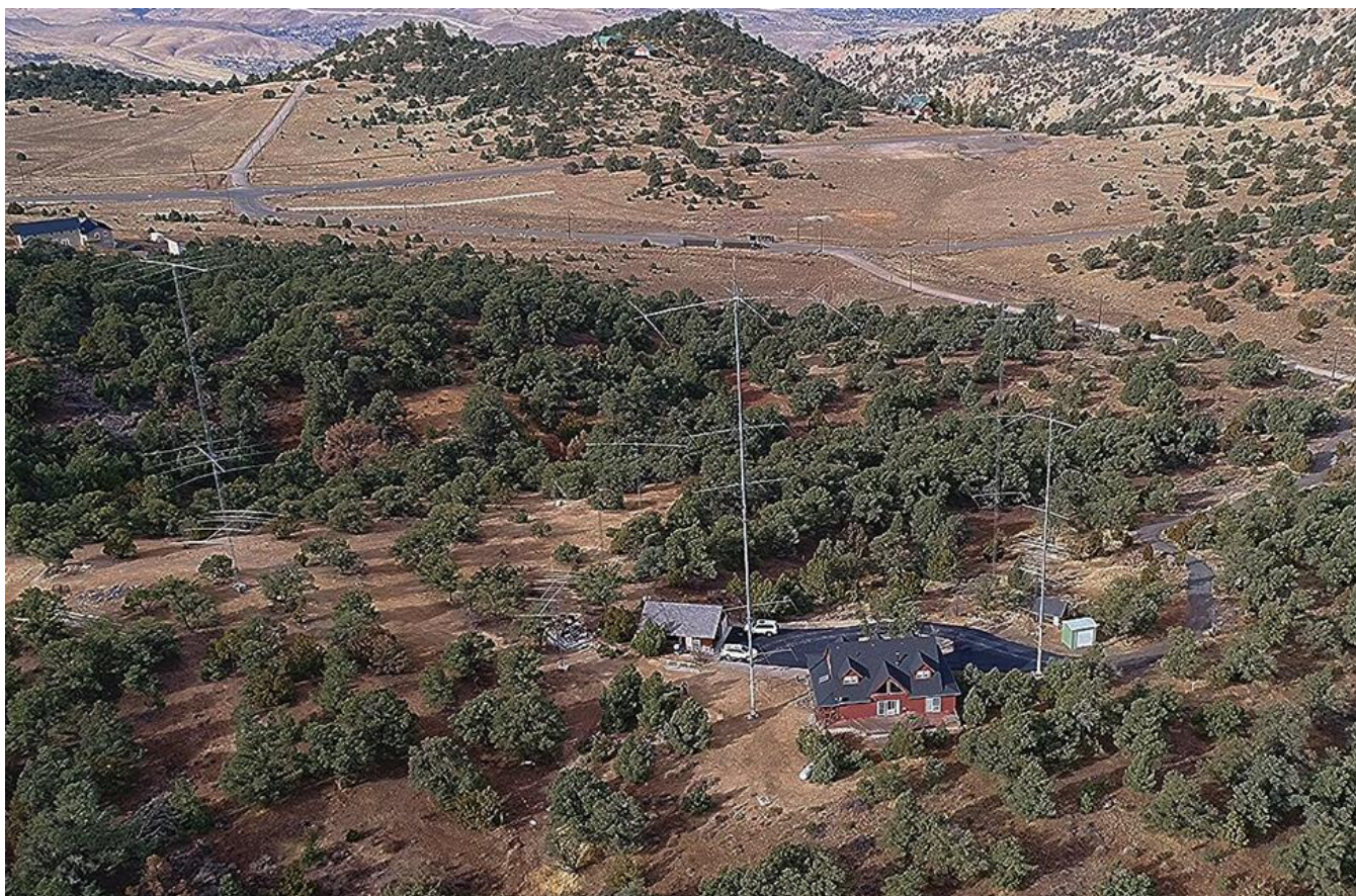
A drone view of the station, looking to the west at the Sierra Nevada Mountains. The centerpiece is a 3-element 80 m Yagi @ 175 feet
