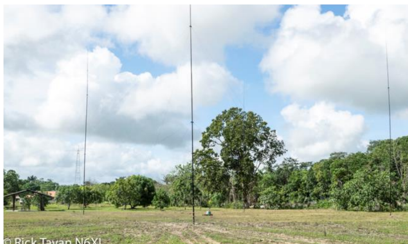
The 80 meter four-square antenna. N6XI photo.
