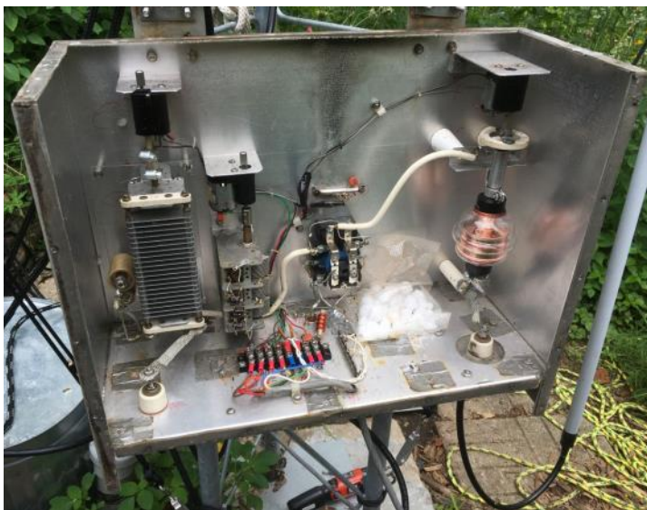
Inside the shunt feed box at the base of the new tower
