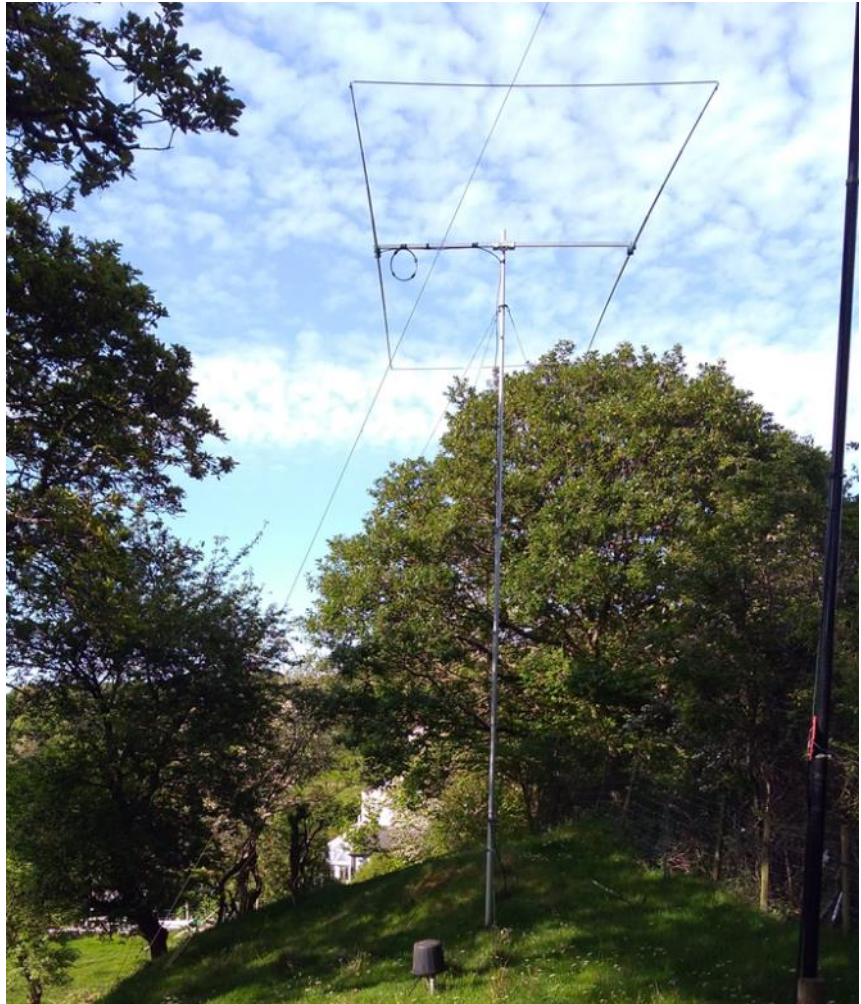
Photo 2 – Moxon nestled amongst the trees with the 20m vertical on the right. Steep slope on the left towards the west. The up-turned bucket is protecting the remote antenna switch.
