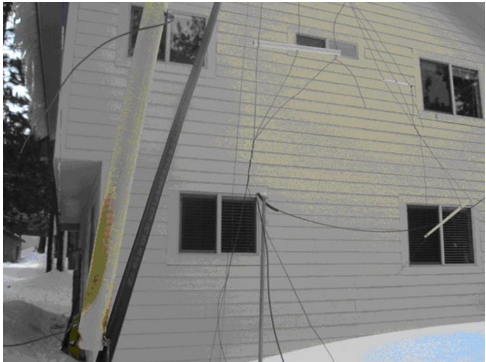
Winter antenna damage at W6SX
