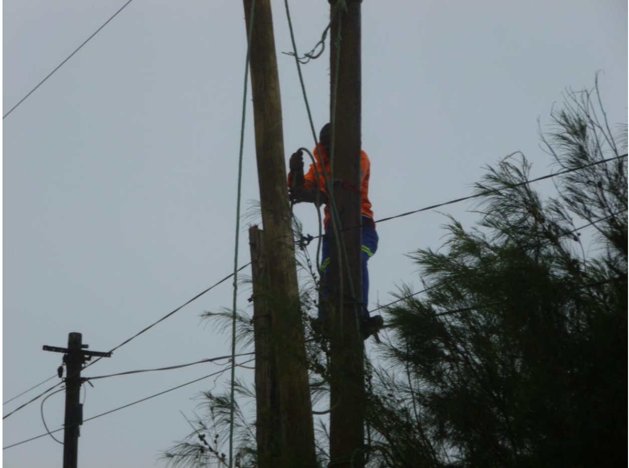
Power company men replace the burned pole with a different wooden pole and move the wires over to the new pole.
