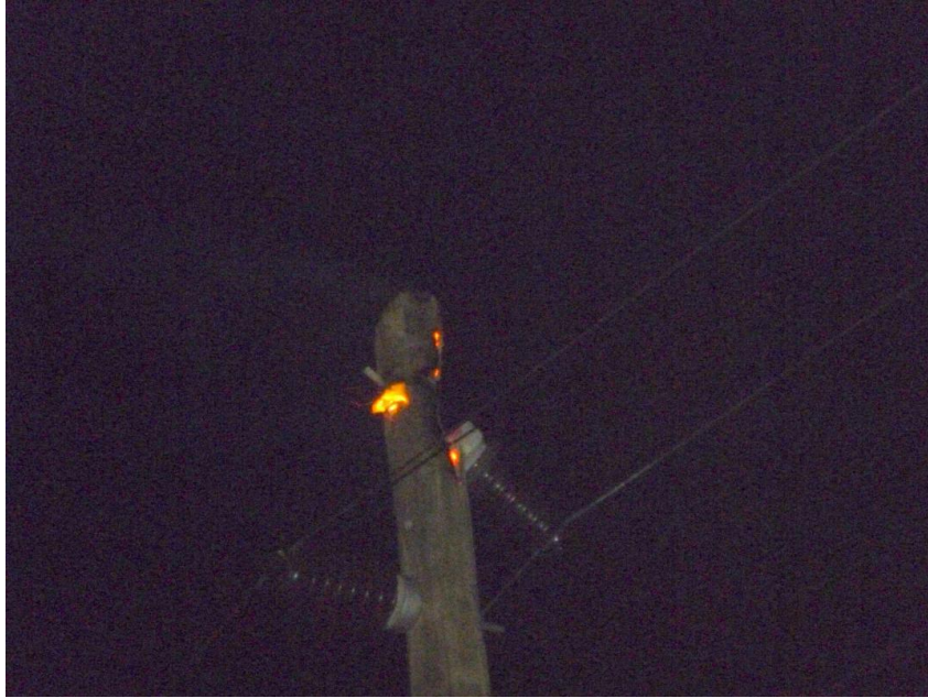
The power pole on fire near the top.
