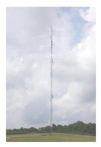
Over time, the antenna farm has grown to a second tower (80') and 4-element yagi's for 10, 15 and 20. The original 100' tower has three tribanders (bottom two fixed on EU) and a 2-element 40 at 100 feet.
